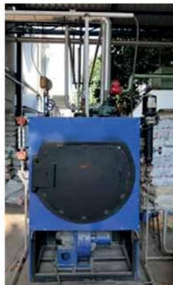
Biomass briquette boiler installed at AGL in FY 2019 (©ABFRL)
