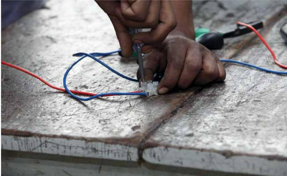
Replacement of splice joints with wire connectors significantly reduces electrical-fire risk (©Sarika Gulati, SEEDS)
