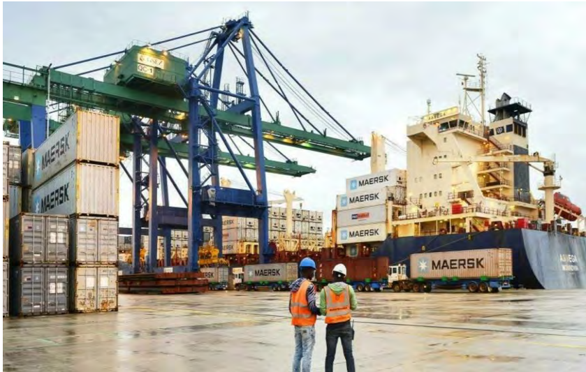
New Owendo international port (NOIP)
