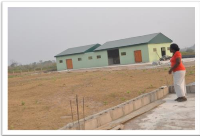
Area view of Psaltry International Limited during construction
