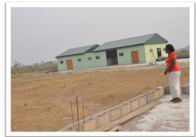
Construction of Starch factory in 2012
