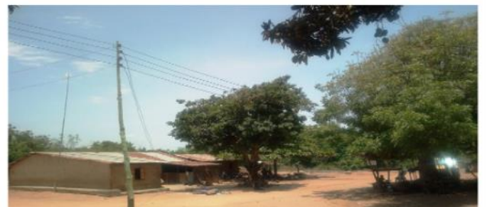
Electricity supply to Wasimi and Alayide Communities.
